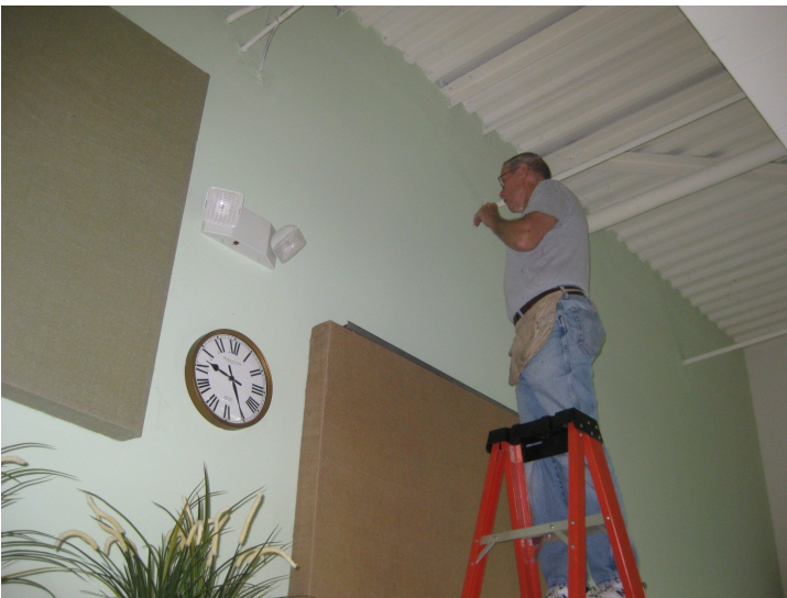
Next, the frame is fitted with a special type of fiberglass designed to absorb sound. You might notice that the fiberglass does not completely fill the frame – there is a bit of an air-space between the fiberglass and the wall which helps absorb the echoes.
